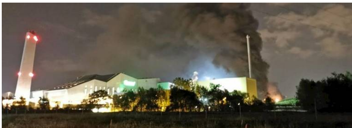
A fire at a waste processing plant in Hengelo, the Netherlands, is probably due to a short circuit (2018).
