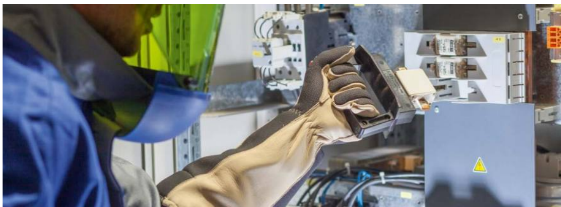
Safely removing NH fuses
